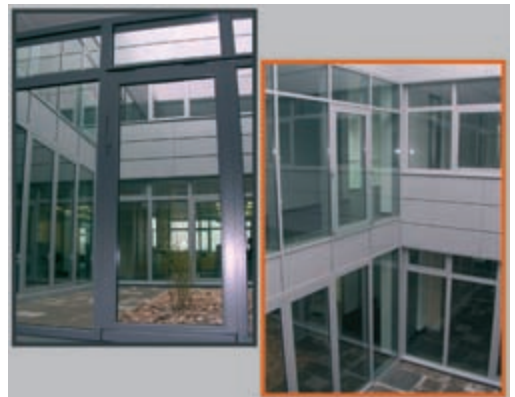
TIGER facility in the Czech Republic coated with chemically crosslinked fluoropolymer powders
